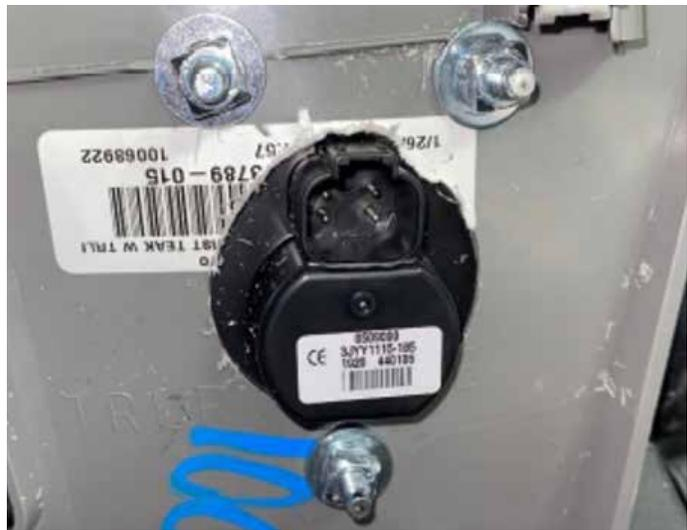
Mount controller on panel using corresponding screw set
